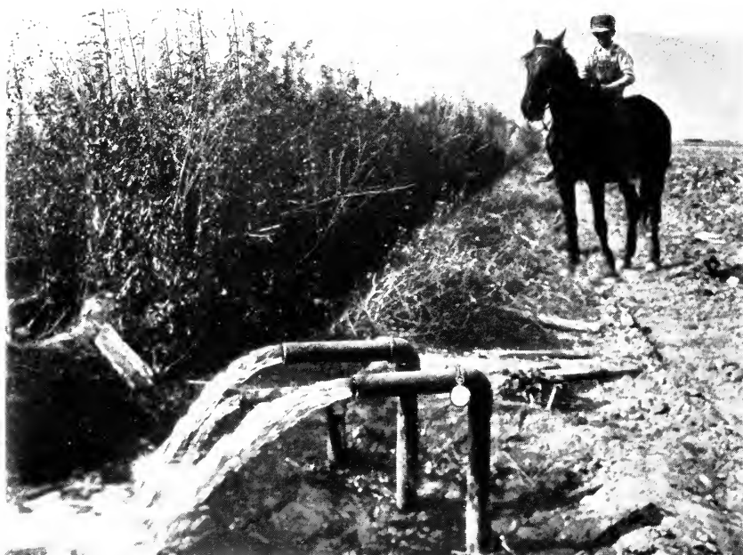
Figure 7. —Artesian well. Water flowing through porous strata is forced to the surface by the pressure of a distant underground reservoir at a higher level.
